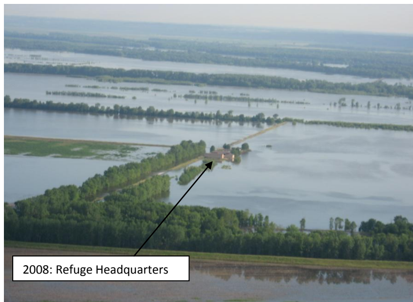
2008: Waters overtop west berm near refuge headquarters and flow towards the town of Annada
